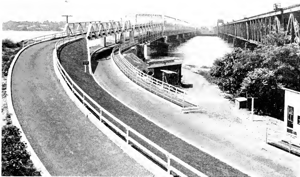
The old Susquehanna River Bridge on U. S. 40 which was double-decked in 1926.
